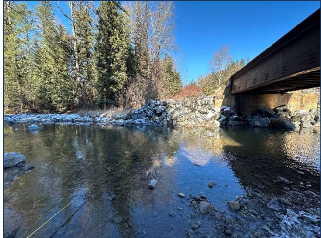
Figure 11: Morrissey Creek hydrometric site (MOR001), across stream from river left.
