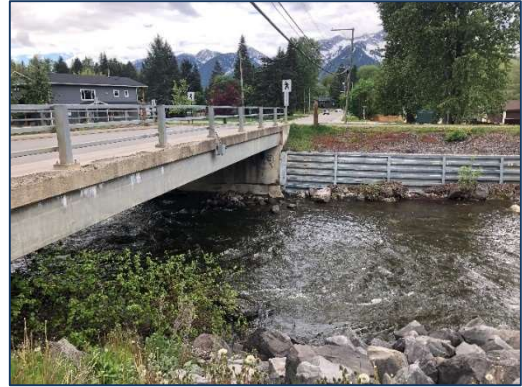
Figure 4: Coal Creek hydrometric site (COL006), looking across stream from river
