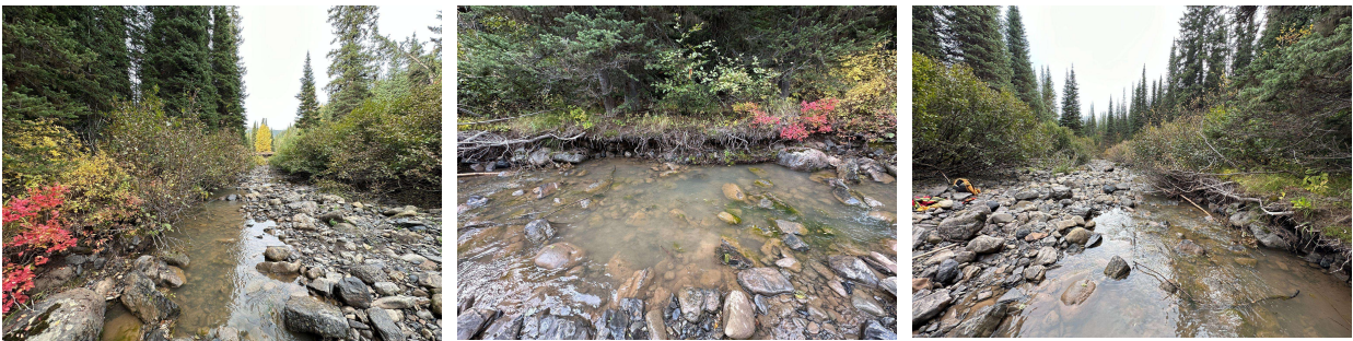
Figure 14. MOR002: upstream, across the stream and downstream.
