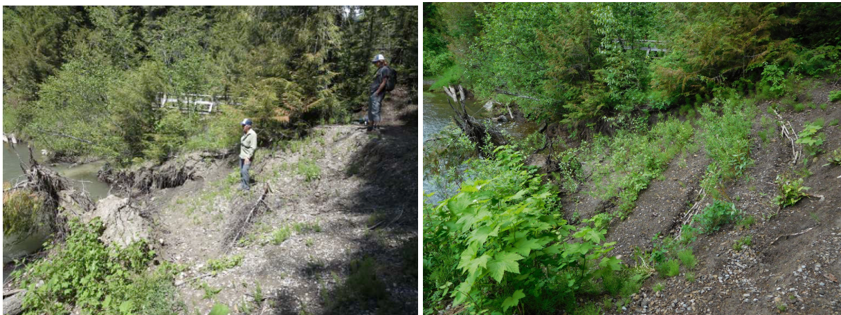
Lizard Creek slope failure adjacent to hiking trail (left 2014) and 3 years after ERA's rehabilitation (right 2017)
