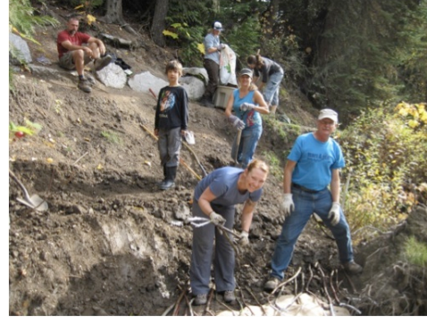
Figure 15- Field crew installing live cuttings
