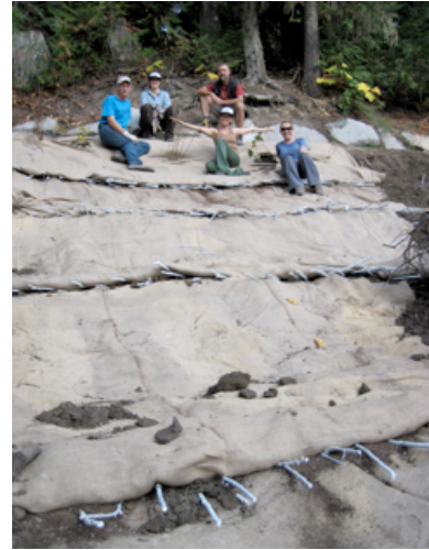
Figure 17- Completed project at Site 2
