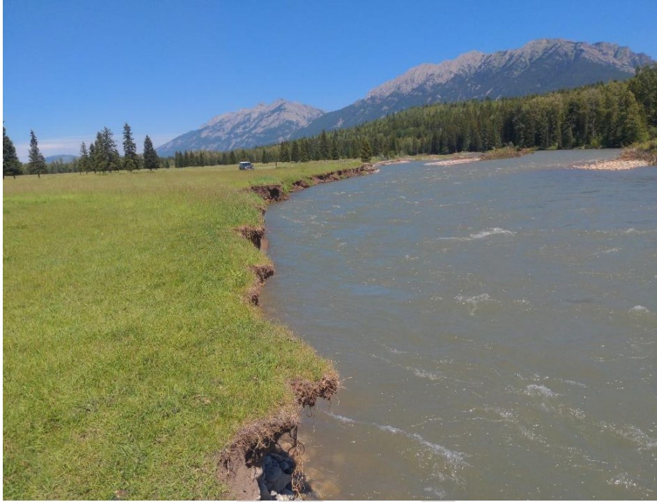
Figure 3. Private property site demonstrating low bank stability and exhibiting no woody vegetation and a strong need for restoration.
