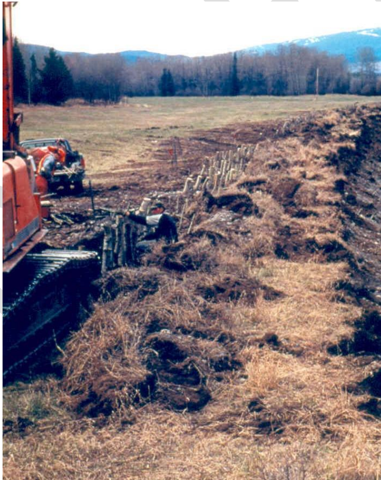
Figure 6. Live palisade method used for streamside restoration. Image shows work conducted by Polster Environmental Services along the Bulkley River (Polster, 2005).
